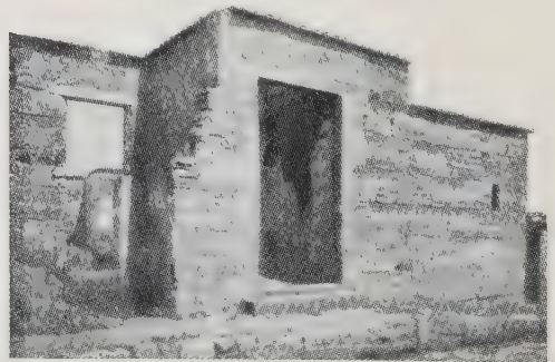
Façade of House of the Surgeon today
